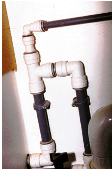
A number of snap-together systems that use O-rings for sealing are neat-looking and quick to install. This is a New Zealand-made system.
