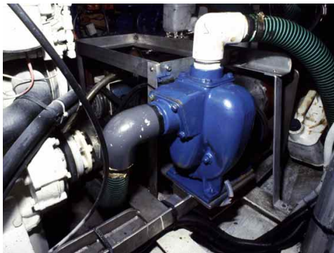
An engine-driven centrifugal pump by Tecumseh. This is the ultimate damage-control pump. It will pass large bits of debris and can pump 200 gpm (775 liters per minute).
