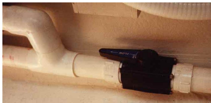
PVC pipe and fittings work very well for both fresh- and salt water and for toilet plumbing. The variety of fittings available allows all sorts of creativity. White plastic typically denotes schedule 40 pipe, while gray fittings are usually schedule 80 (which is much heavier).
