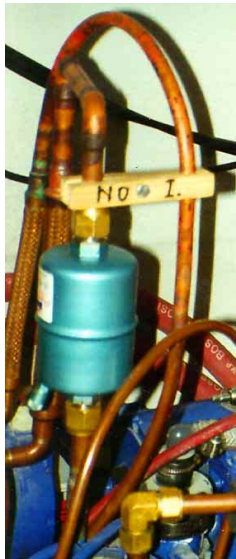
Vibration in fridge fittings causes more problems than anything else to do with these systems. Generous loops of copper, with secure clamping to limit harmonic vibration, helps (left photo).
