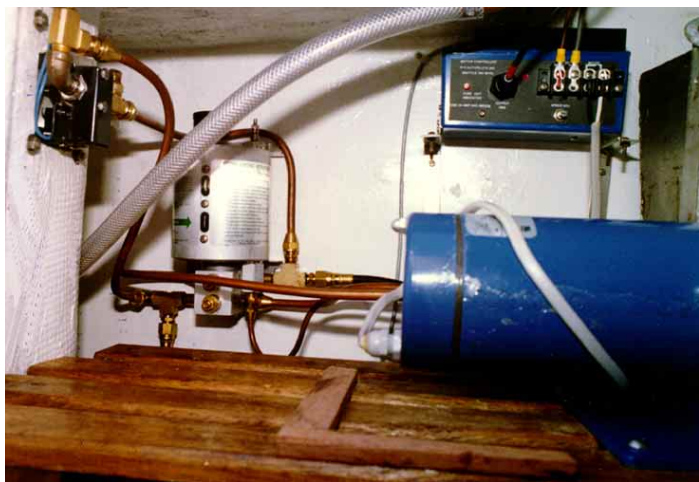
A 1/4-horsepower WH pump set. If copper tubing is used, flares must be carefully made, the tubing should be supported, and the best-quality hydraulic tubing (not refrigerant tubing) used. We prefer to use high-pressure hose or stainless-steel tubing in systems where the operating pressure are likely to be high.
